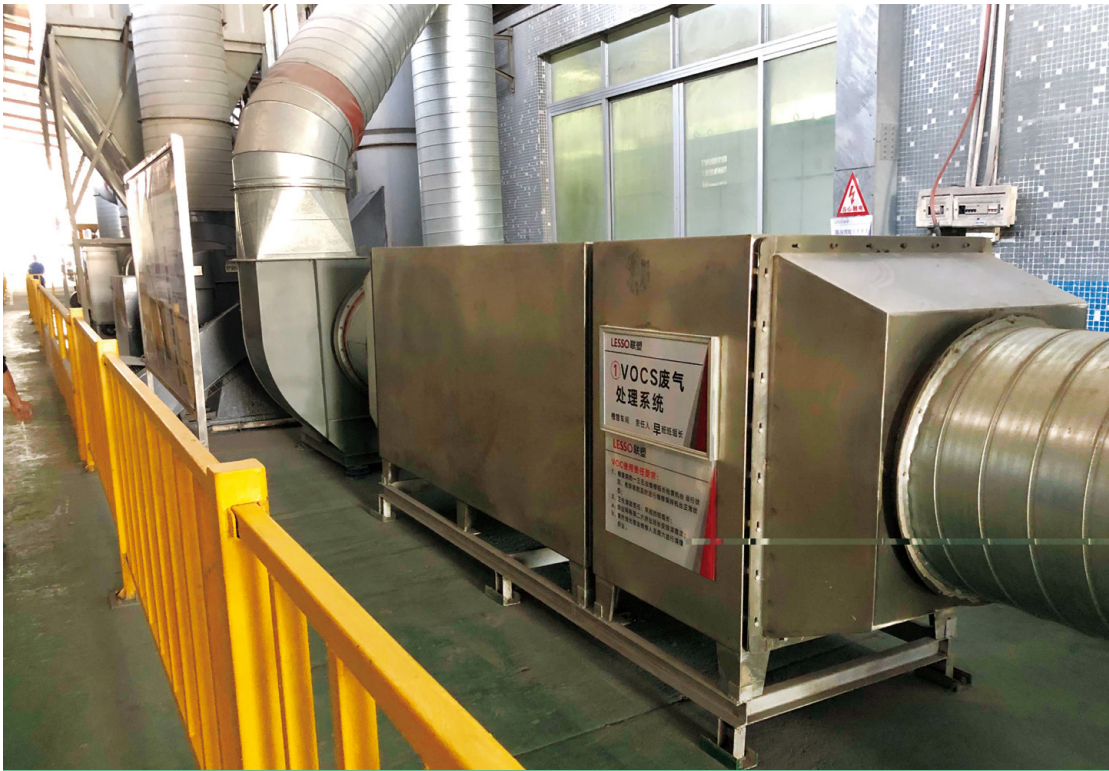
VOC exhaust treatment and environmental protection system VOC
